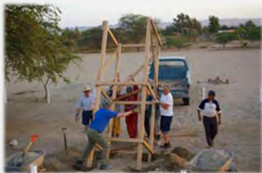
TeamWorkers building children's playground at Betel (Bethel) Bible Camp
