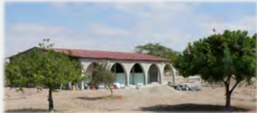
New auditorium at Betel (Bethel) Bible Camp – June 2009
